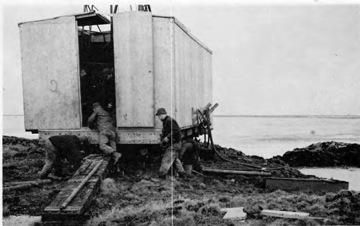
Core drilling at the Simpson Camp.
