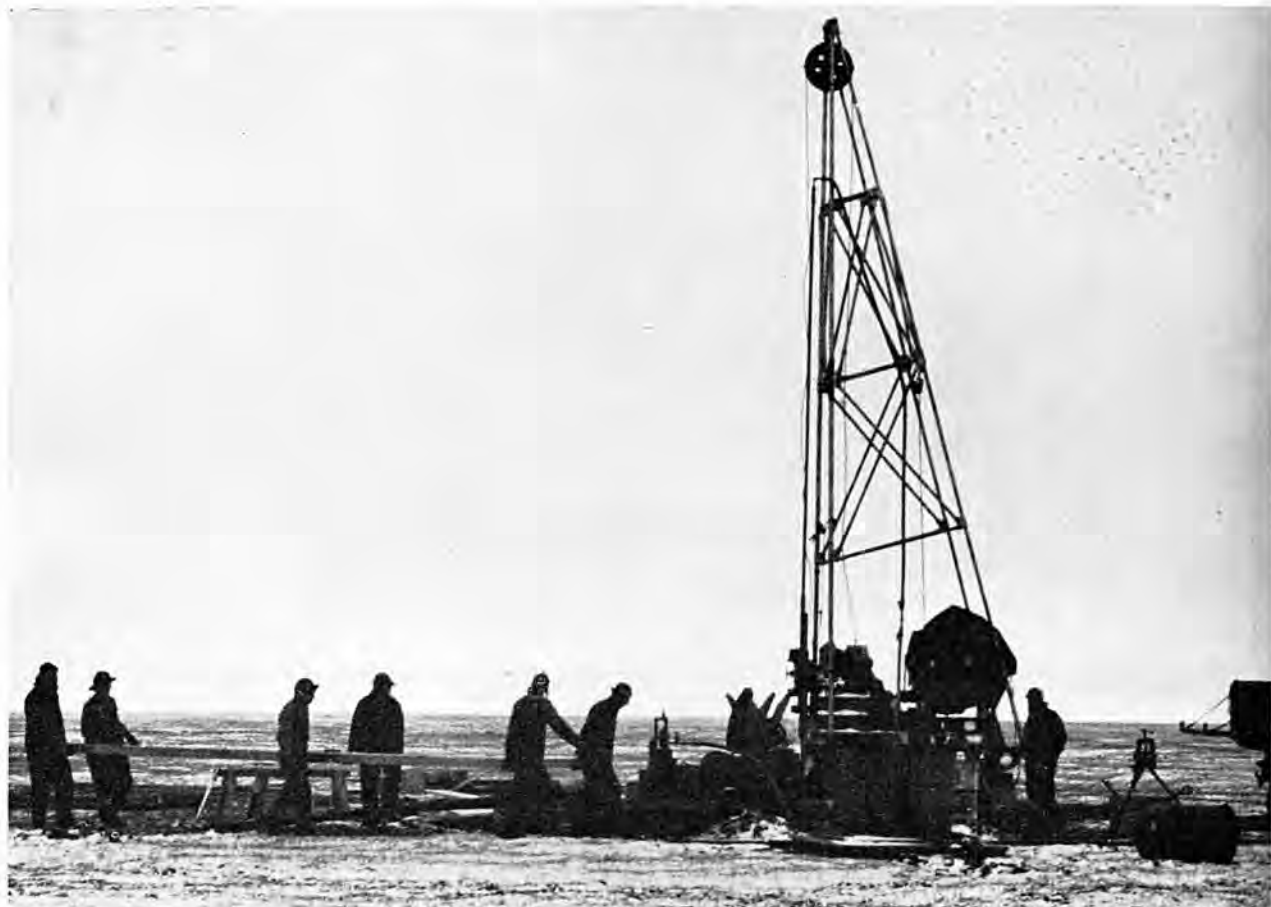
SEABEES AT POINT BARROW Members of the 1058th Detachment setting up the core hole rig for test hole No. 1
